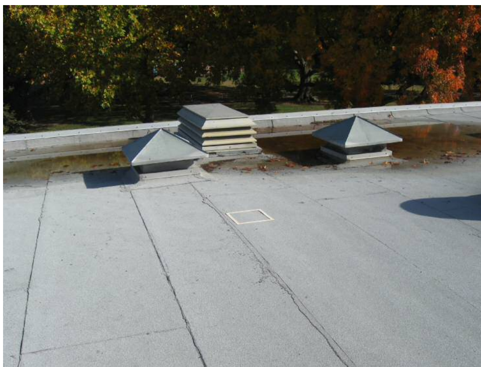
Roof - sampling surface of roof in middle of roof "field"
